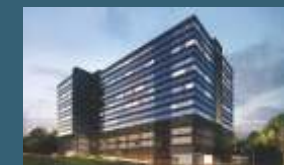
SEZ at Blue Ridge, Pune
